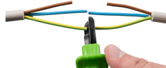
Cut out the damaged areas in the copper and disconnect all other conductors. For damaged areas between 1 mm and 30 mm, at least 30 mm of the damaged conductor must be removed. Tip: A connector (approx. 30 mm long) can be used as a length guide.
