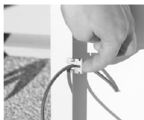
1 Position grounding clip with electrical cable inserted in it and the bottom of the part outside the frame
