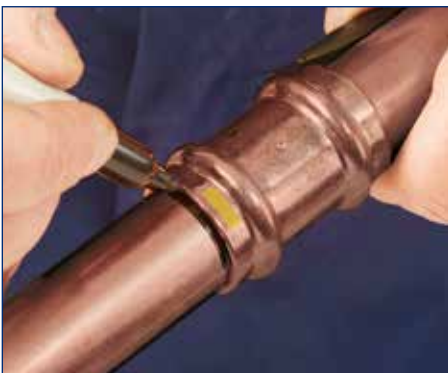
4. Assemble & mark the insertion depth
